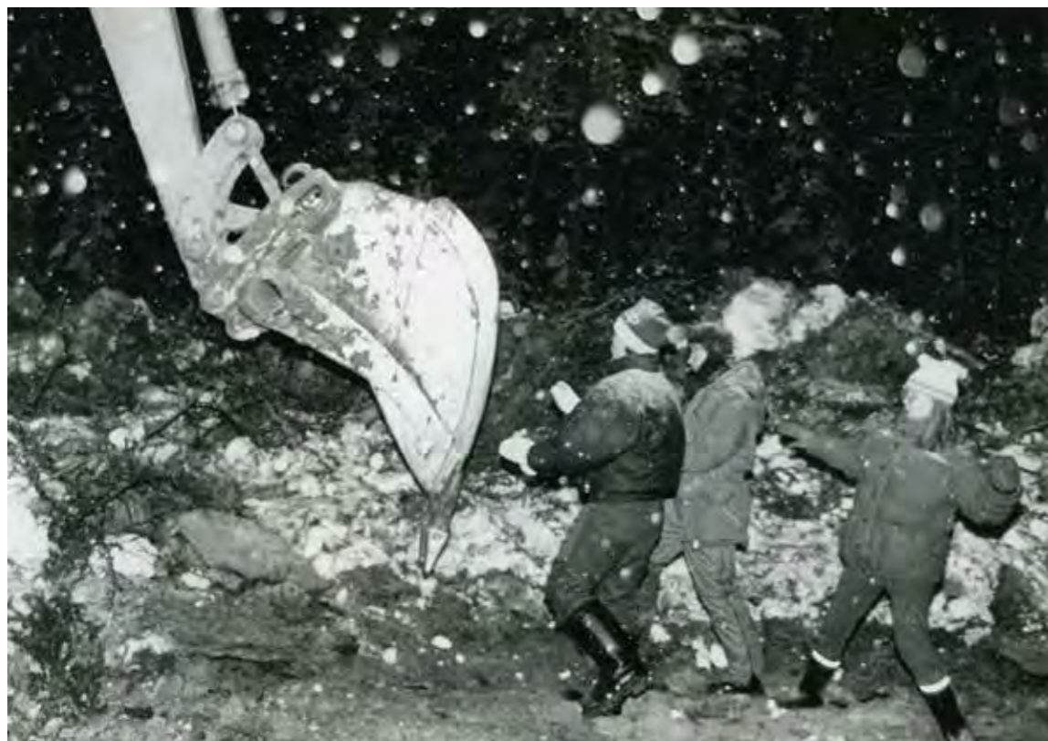
◆ The 'forest wars' started in the 1980s. Here, three young activists confront an excavator at Lake Jerisjärvi during the Pallas–Ounastunturi road dispute in 1991. The Finnish Nature Association Collection, Lusto.
