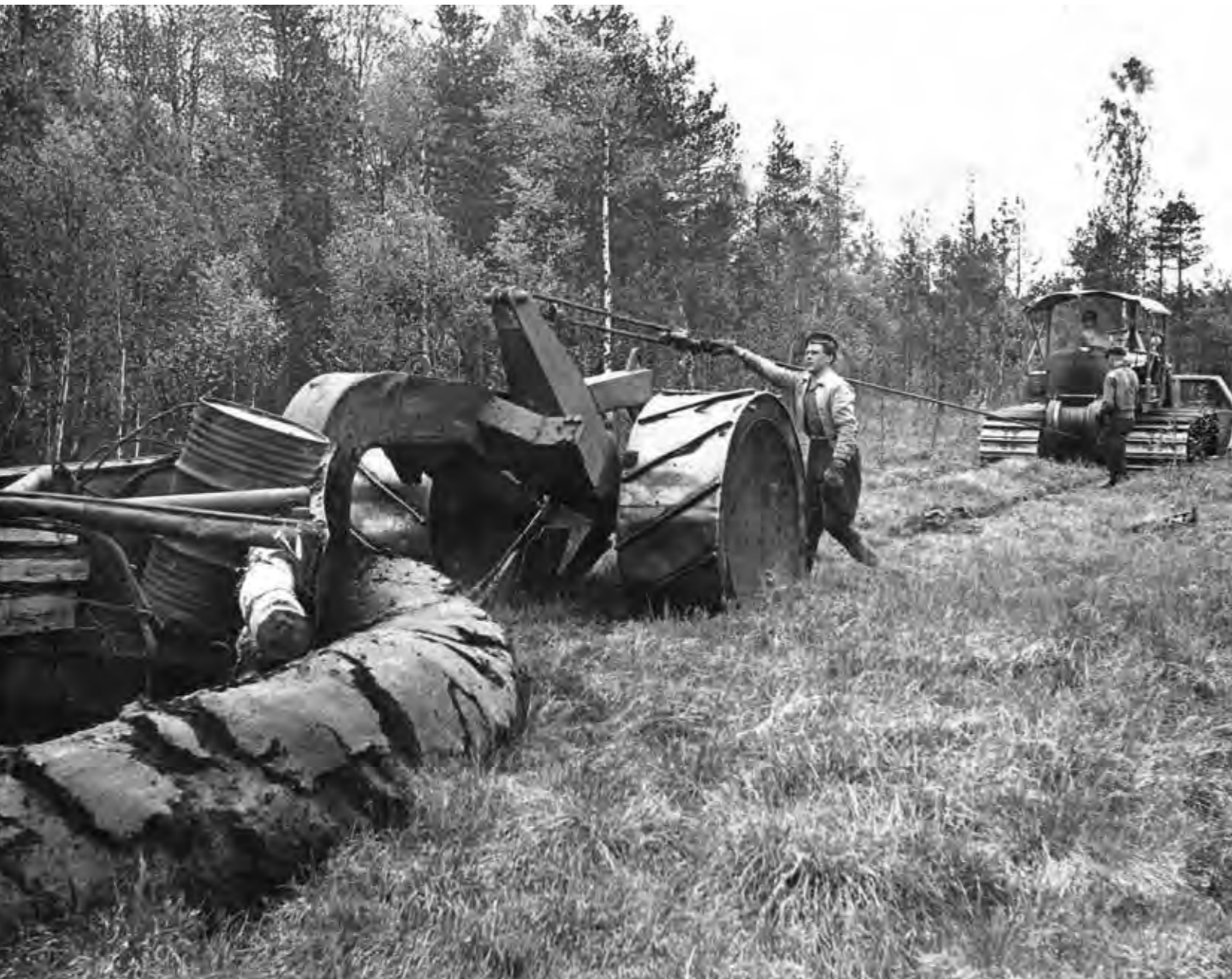
◆ Mechanical draining of spruce and pine mires and swamps began in the late 1950s. The aim was to increase timber volumes and secure the supply of raw material for the forest industry. Heavy draining ploughs pulled by crawler dozers cut straight ditches at regular intervals. Metsätaloudellinen Valistustoimisto, the Finnish Forest Association Collection, Lusto.
