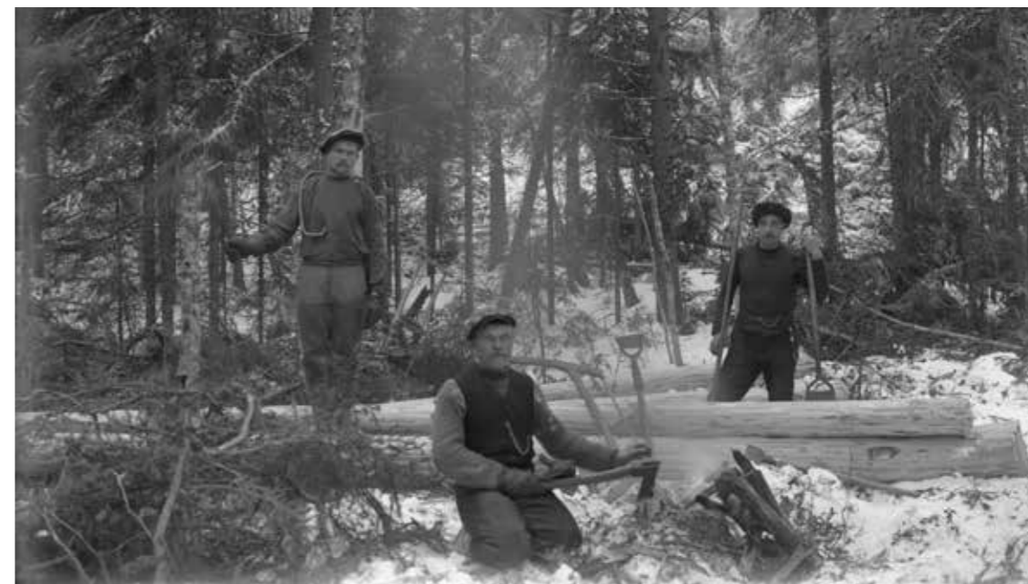
◆ As the forest industry expanded, logging operations spread ever further inland. In the Virrat region, forests were left in poor condition. In this image, men are seen lopping branches off spruces with axes and debarking logs with bark spuds in a forest in late winter. Matti Luhtala, the Vapriikki Photo Archive.
