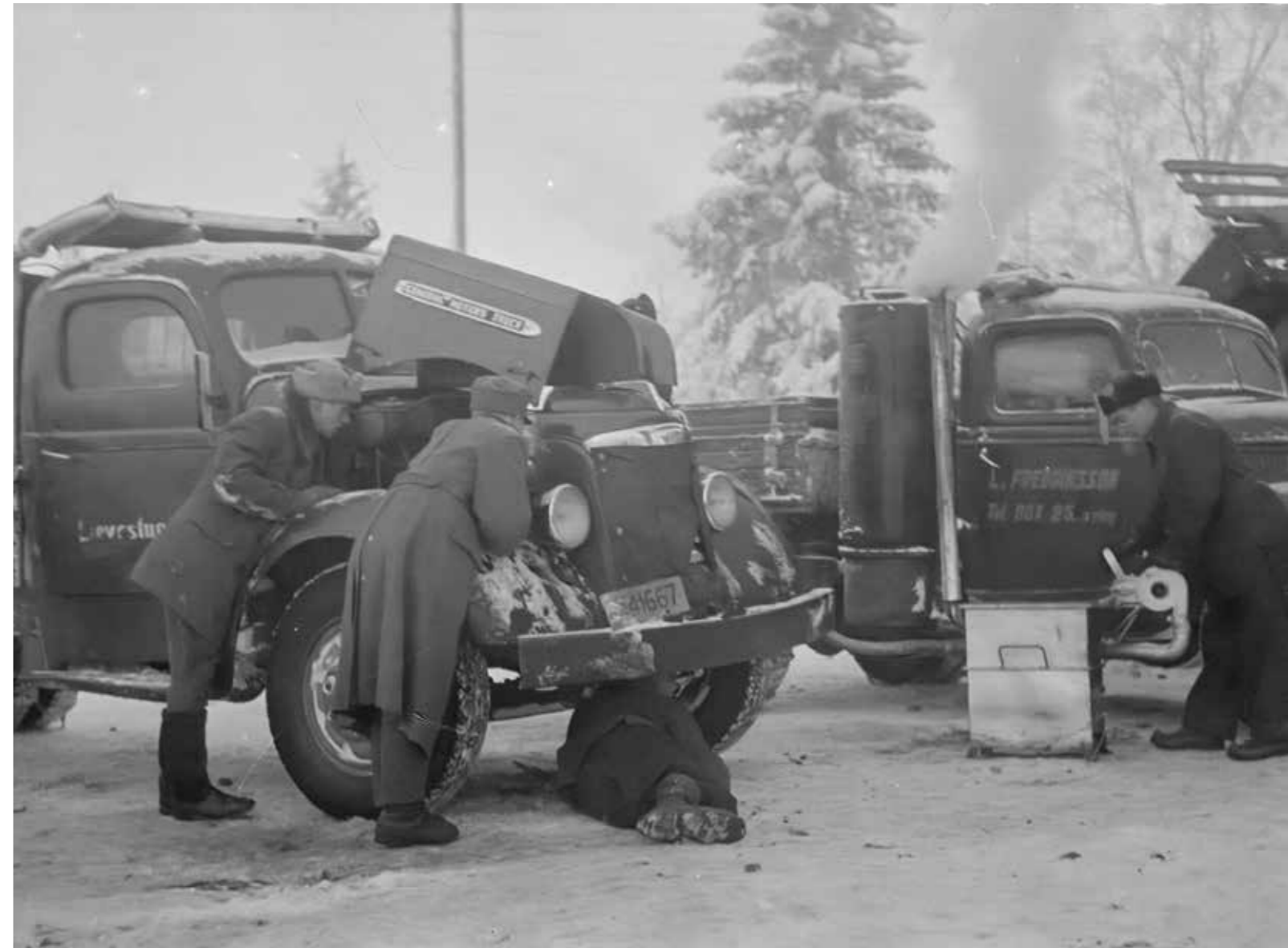
◆ Liquid fuels were in extremely short supply during the war, so wood-gas generators were installed on passenger cars, lorries and buses on the home front. The engines of these vehicles had to be preheated during periods of severe frost. The Mänttä Club served as a military logistics training centre during the Continuation War 1941–1944. SA-kuva.
