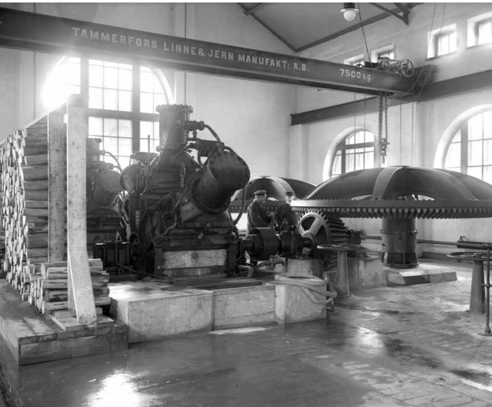
◆ The forest industry has been extremely important for Finland's national economy. The Finland of the 1920s and 1930s has been called 'the Forest Republic' as more than 80 per cent of the value of its exports was generated by forest industry products. Pictured is the mechanical pulpwood mill at G. A. Serlachius Ltd's Tampere factory in 1908. The Vapriikki Photo Archive.
